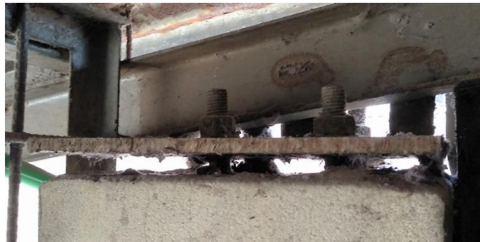
Rafter-column Connection
