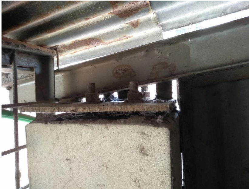
Significant gap observed between steel baseplate and RCC column.
