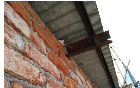
Non-engineered connection
