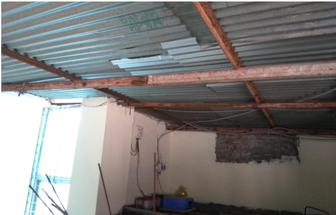
Light weight roof supported on brick wall
